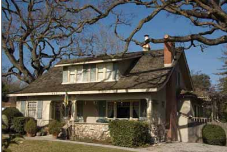
1. Side Gable Massing with shed dormer and integral porch under swayback roof
