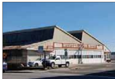
7. Saw-tooth warehouse building
