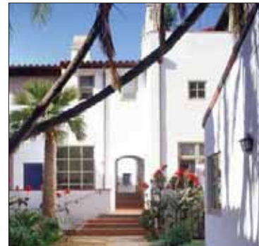
Illustrative Photo Courtyard with zaguan linking two courtyards
