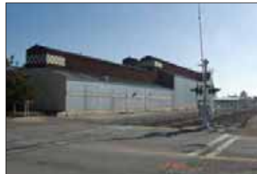
5. Industrial warehouse building with roof monitors
