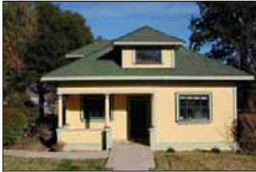
2. Hipped roof form, integral porch and front dormer
