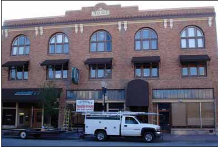
1. Three story brick building with five bays and three shopfronts
