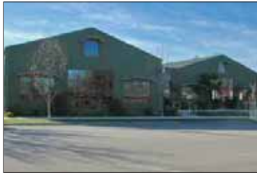
4. New warehouse building with office uses
