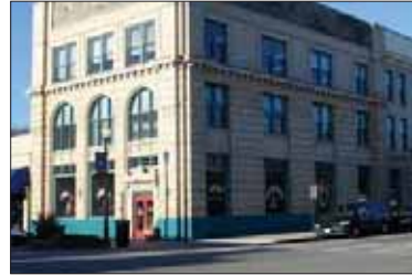
4. Three story masonry building with heavy pier accents
