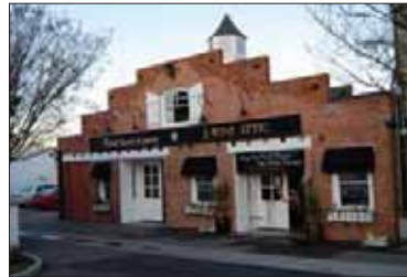
3. Single story gable end with stepping brick parapet
