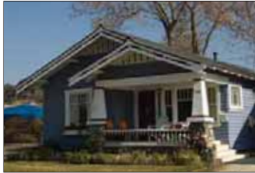
3. Gable end with front porch
