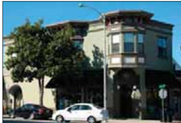
6. Victorian two story building with corner chamfered bay
